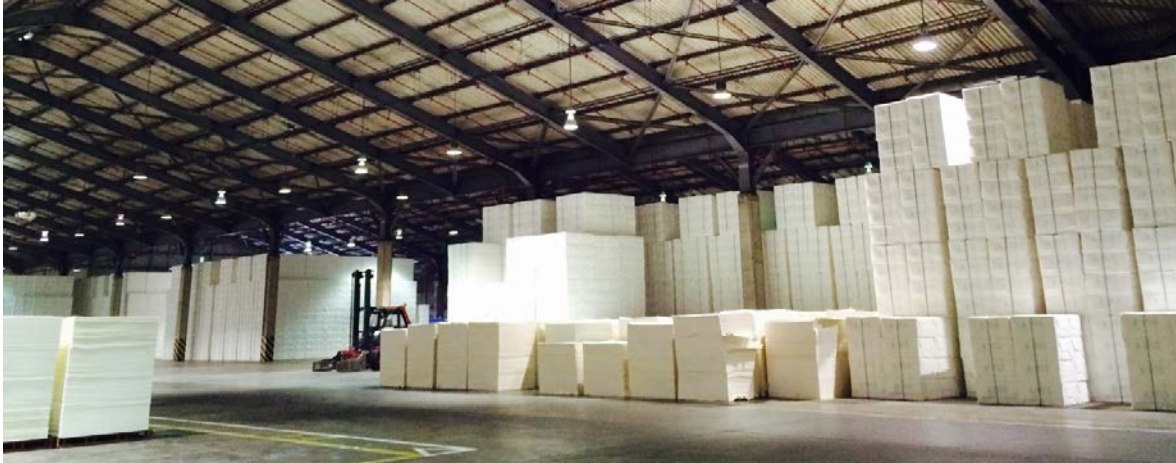
Figure 8. CMPC Plant Nacimiento, Chile. Cellulose pulp storage for export.
