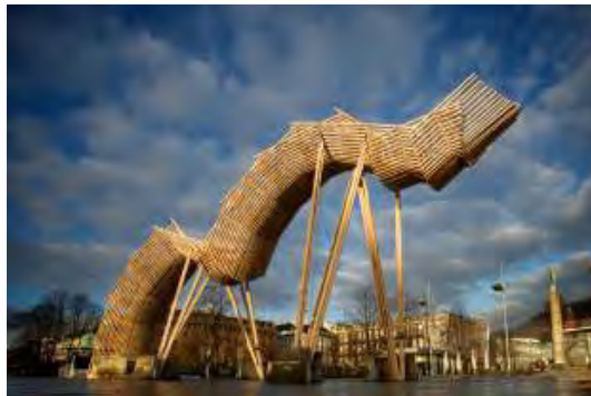
Image 9. Hunter First, we set up a solid anchorage on the ground, and then we built sideways as far as we dared. Then to continue supporting the structure with posts.
