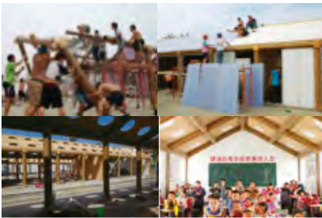
Figure 5. Chengdu after-quake paper tube school by Shigeru Ban et.al (from Shigeru Ban Architects)
