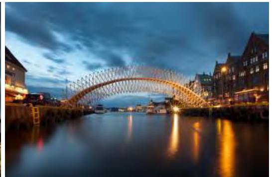
Image 10. The Bridge Our point of departure was again to challenge the constructive properties of wood – structurally and visually. In constructive terms, it was tempting to test a form based on the wood's ability to withstand bending as well as pressure and span forces.
