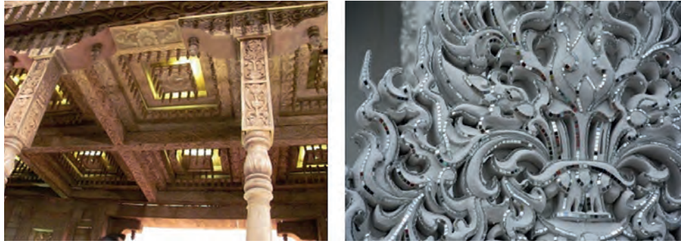
Figure 18 & 19. Use of detailing in materials: wood, PoP.
