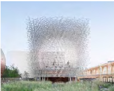
UK Pavilion, Milan Expo 2015, Italy
