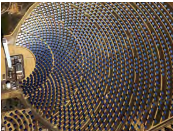
Image 4: Seville solar plant
