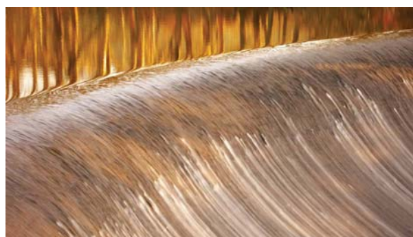
Figure 4: Upper overflow - Abbeystead Dam
