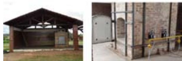
Figures 11 and 12 – Annex and gas kiln in the Center for Craftwork
