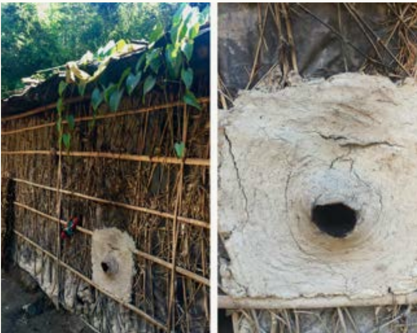
Figure 6. The indigenously built chimney on the mud wall (Photographs ©Indrajit De & Saumya Pande)
