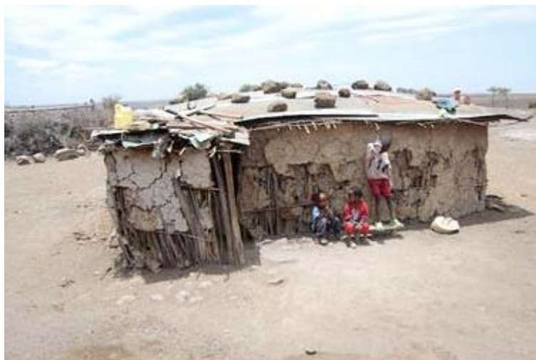
Figure 3: Typical BOP housing in the Kenyan steppe
