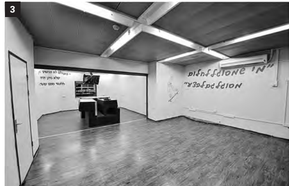
Figure 3 The youth center before renovation.
