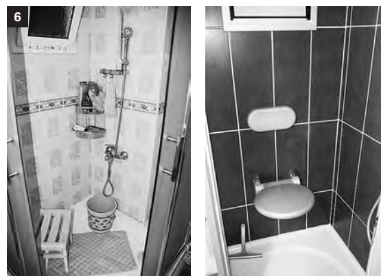
Figure 6 Traditional ways of bathing. On the left; a plastic stool to sit on, a plastic bucket to store the water and a plastic bowl to pour the water in the shower cabin. On the right; a foldable seating unit mounted on the shower cabin wall of a renovated the bathroom (photographed by the author).
