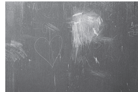
Fig 6: Graffiti imprinted onto the exterior curved walls. Karijini National Park Visitors Centre (photo), Pilbara region, 2001, Architect – John Nicholas. Source: Author.
